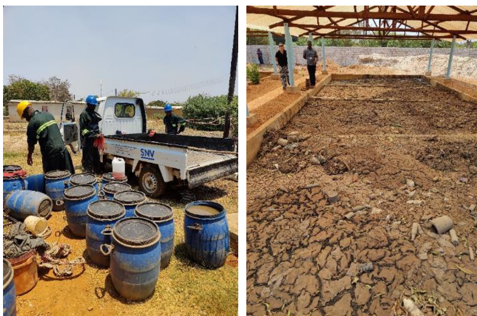
Figure 6 Faecal sludge removal by private emptiers and drying beds in Kabwe, SNV, Zambia
